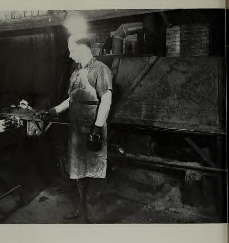
After any remaining babbitt is chipped off with a chisel, the bearing end of the rod is then dipped into a solution of hydrochloric acid. The acid acts as a cleaning agent. The acid vat is under the wooden cover shown at the right in the above picture. Then the bearing end of the rod is dipped into a molten tin or solder shown on the left in the above picture. This solder or tin acts as a flux or bond when the babbitt is cast against it.
